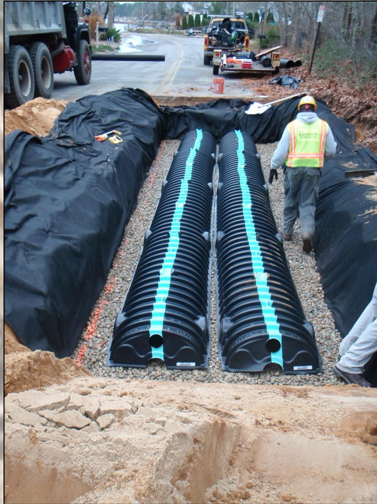
Drainage System #7 – Cultec Chambers
