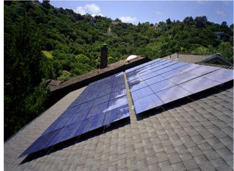
Roof mounted – can be flush to roof pitch, mounted on a fixed rack for proper angle, mounted on adjustable rack
