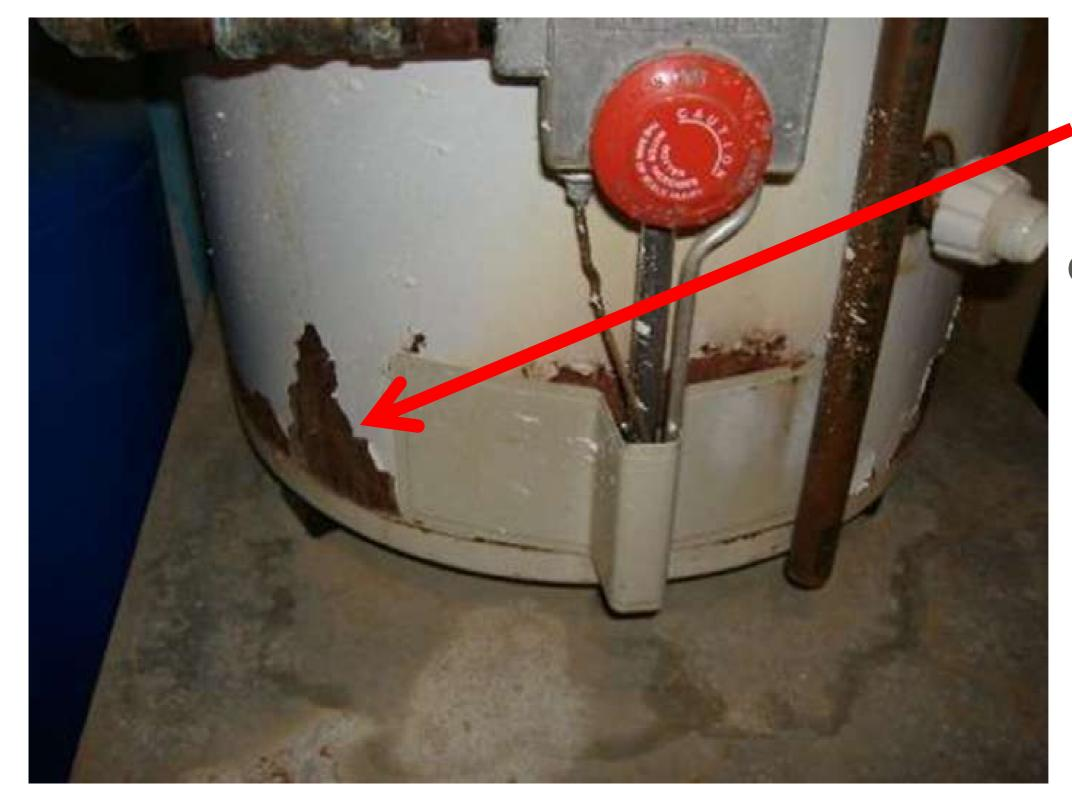
Water Heater starting to deteriorate
