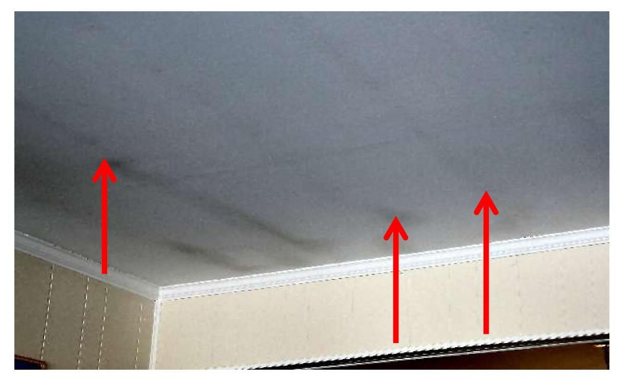
Cold Ceiling (poorly insulated attic) collects moisture and any particles in the air, staining ceilings.
