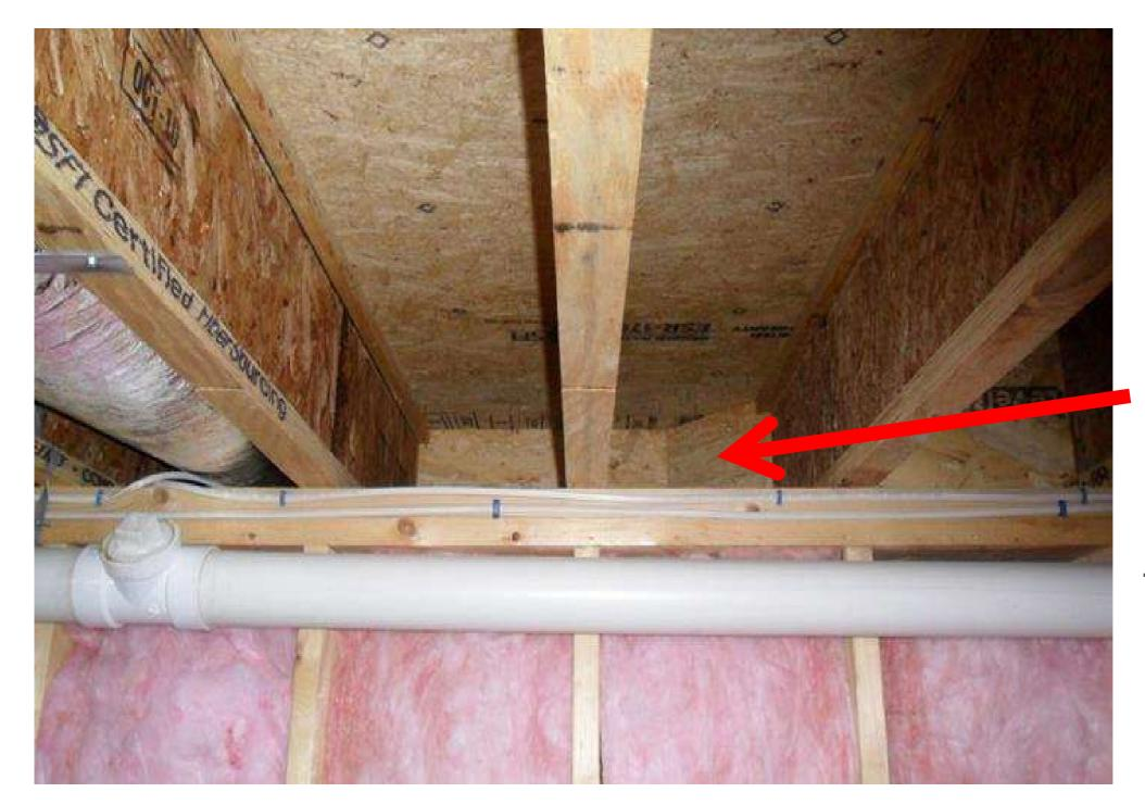
Uninsulated rim and band joist located above insulated foundation walls
