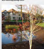
This bioretention pond in Williamsville, Oregon collects runoff from the rooftop, sidewalks and yards. The pond offers valuable aesthetics and wildlife habitat benefits while also reducing stormwater control costs.
