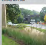
Philadelphians have been extending the use of LID by implementing new policies and demonstration projects, such as this residential bioswale that treats runoff from an adjacent parking lot. The city's use of LID has reduced stormwater runoff volume, saving approximately $178 million in combined sewer overflow costs since 2006.
