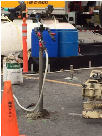
Pumping of diluted SRS®-NR EVO into injection borehole
