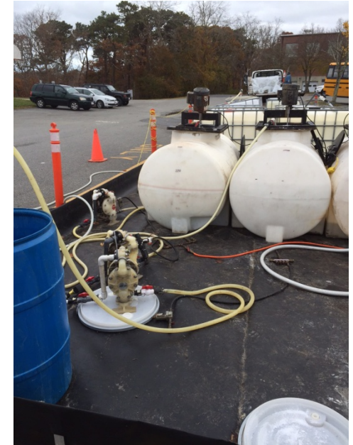
TSI's SRS®-NR EVO diluted with water prior to injection
