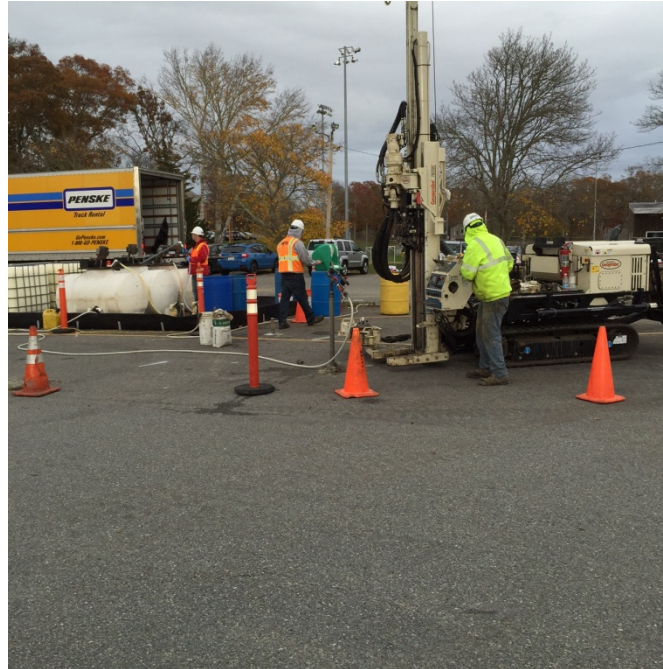
Injection boreholes advanced using direct push drill rig
