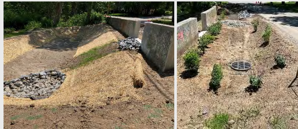
Timberlane Drive Stormwater Retrofit
