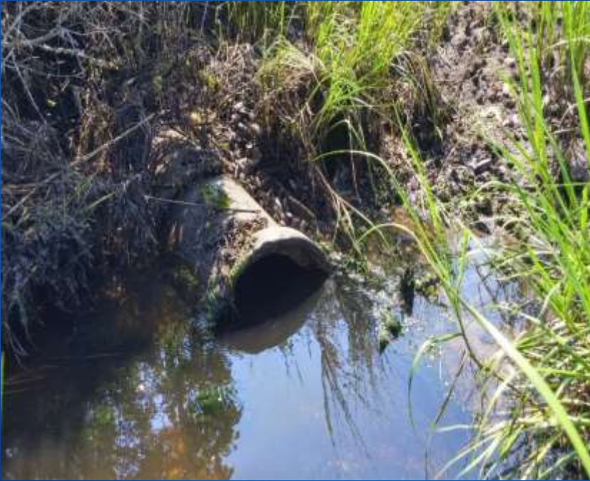
Undersized tidal culverts
