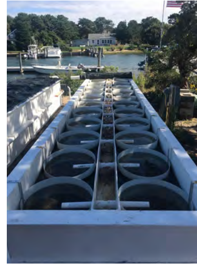
2 Land Based DuraTech Downweller/ Upweller tanks – 48 x 2' diameter silos, 4 pool pumps, plumping, electric $$$
